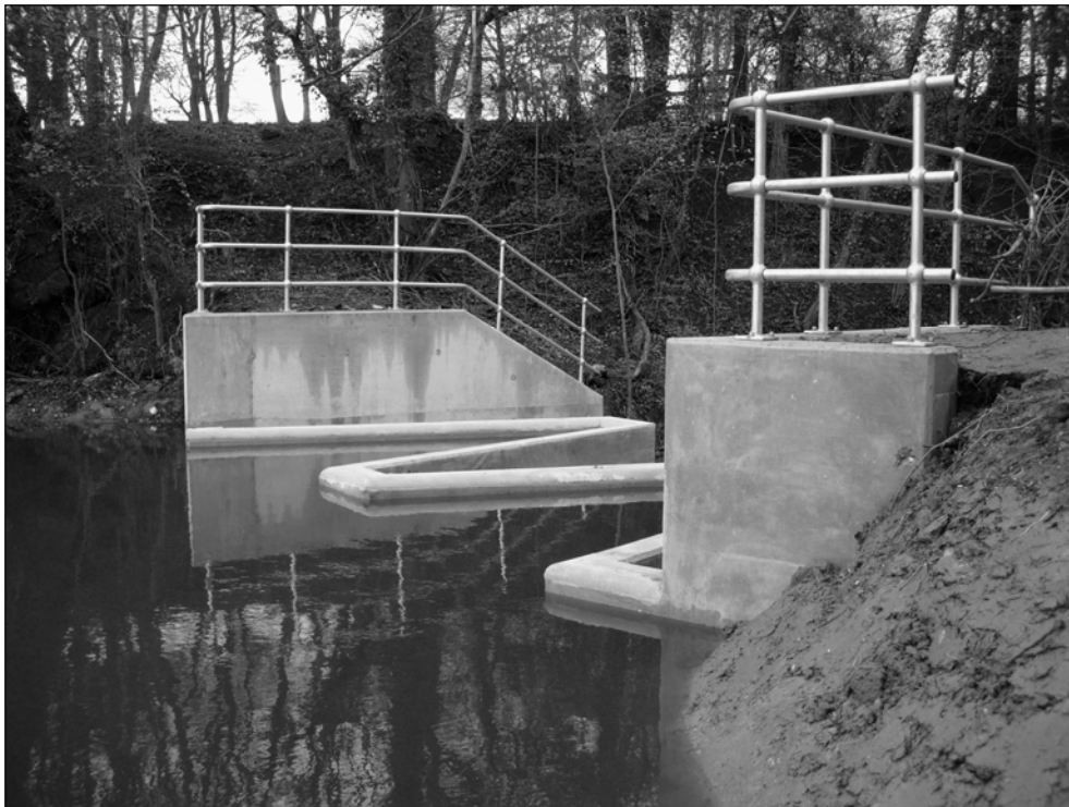
Figure 3. The completed labyrinth weir structure
